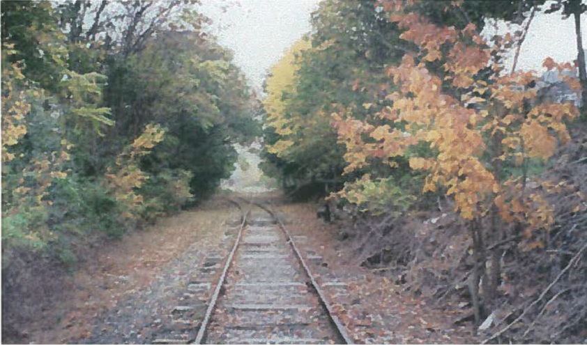
Rail Right-of-Way East of Cedar Street, 2001
