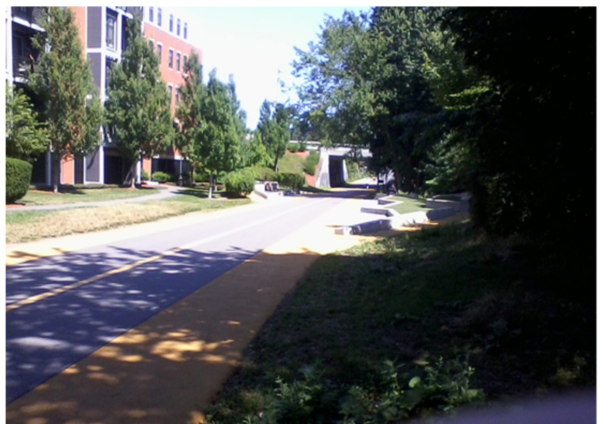
Community Path at Lowell Street, 2020
