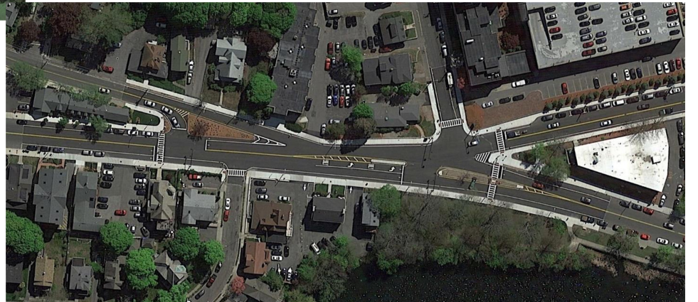
After Reconstruction, May 2016
