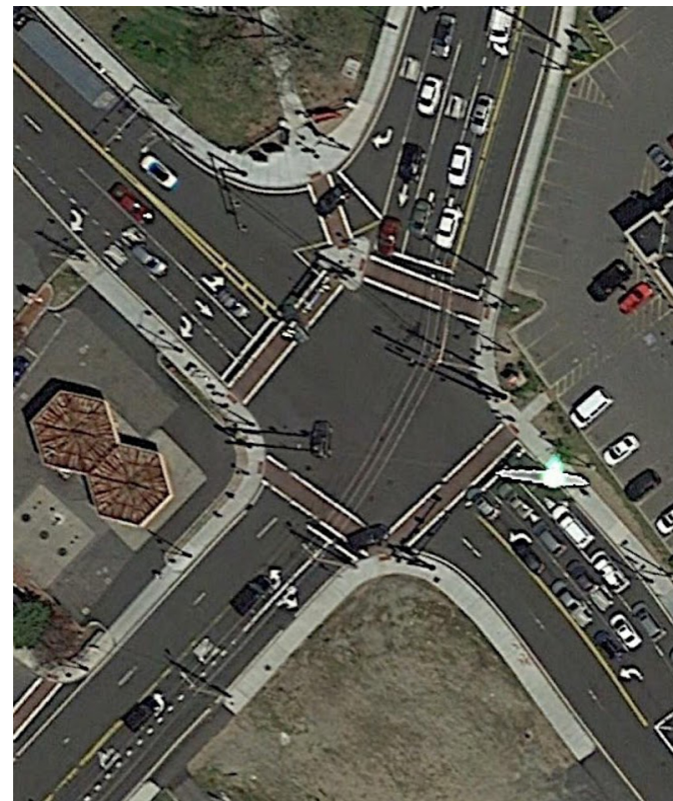
After Reconstruction, May 2016
